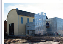
Cultural Centre Proevhallen
