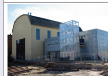
Cultural Centre Proevhallen
